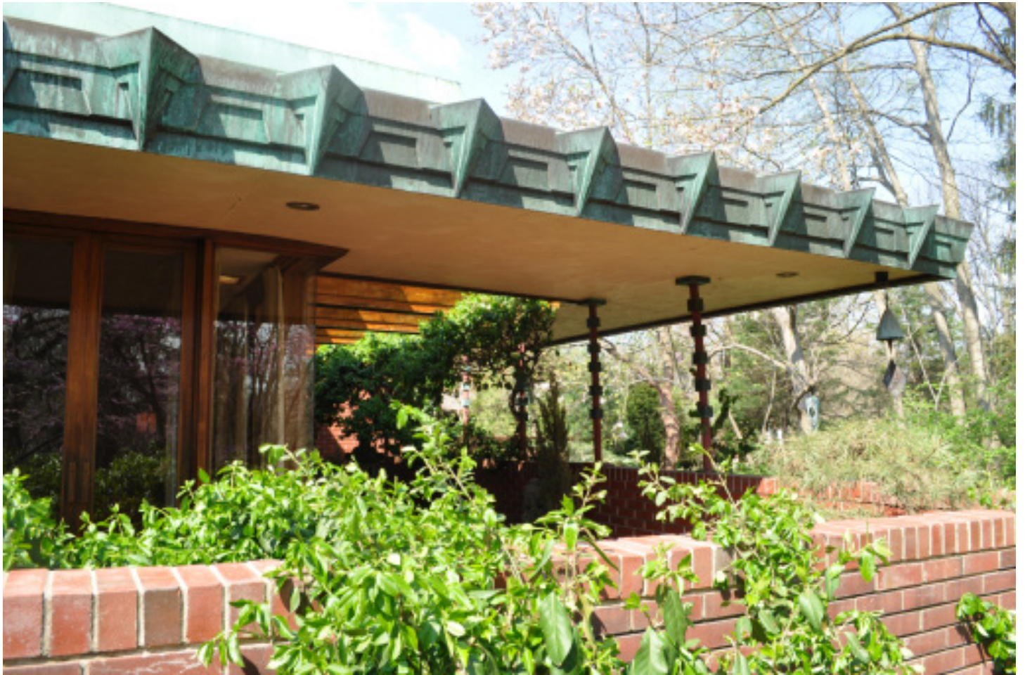
Samara, exterior view of terrace from west, 2012, digital image. Image: April Befort.
